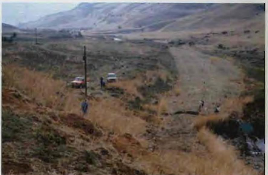
Figure 9: Single Wire Earth Return Transmission line
