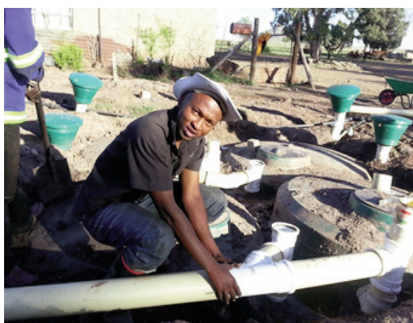
Figure 5: Trainee connecting effluent pipes
