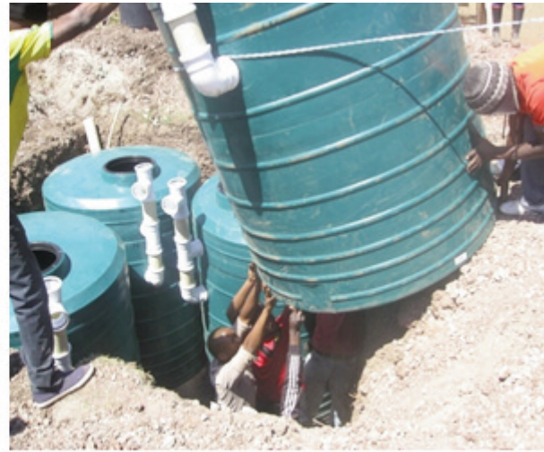
Placing digester tanks in side hole
