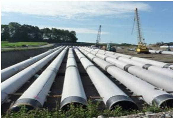
**Figure 7: Surface pipeline compressed gas storage (Bilfinger Industrial Services GmbH (BIS), 2021).**
